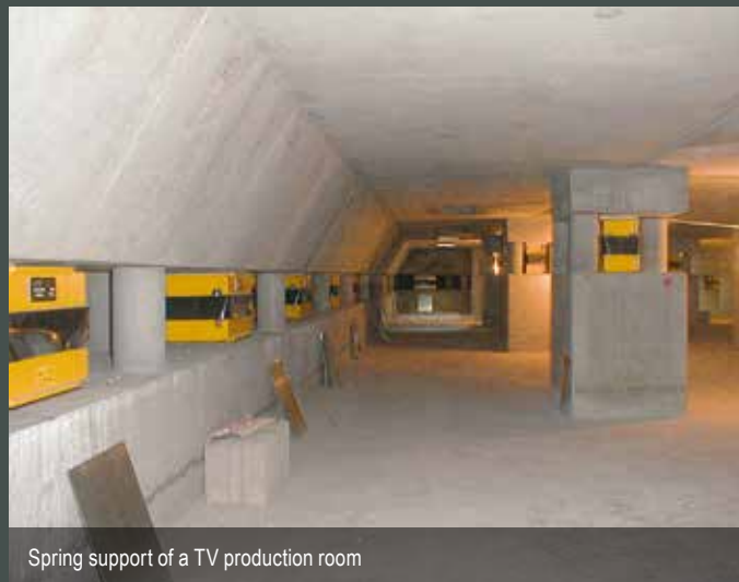
Recording studio with floating floor
