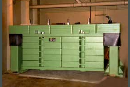
MS "Deutschland" with Tuned Mass Dampers (TMDs)
